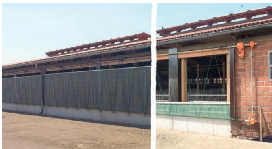
Roller curtain opening from the top to the bottom using the EWA actuator
