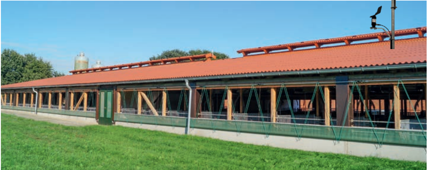
Pig house with open-air run and curtains as protection against the weather
