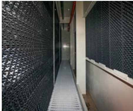
Filter bank (left) and droplet separator (right)
