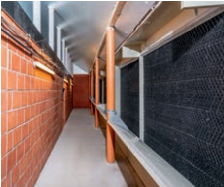
Fans press the exhaust air into the first pressure chamber and then through the plastic filter
