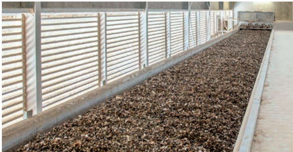
View of the topmost tier with a manure rake at the end to loosen the manure layer
