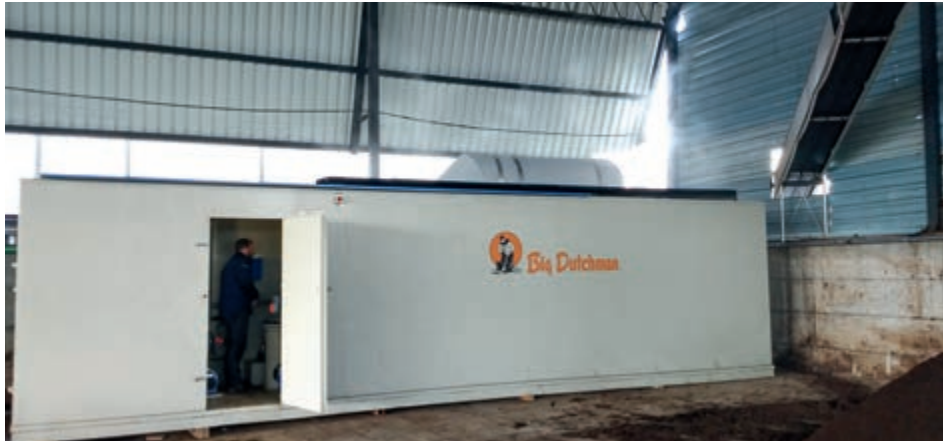
View of the CompoLiner exhaust air cleaner as a complete system ready to be connected
